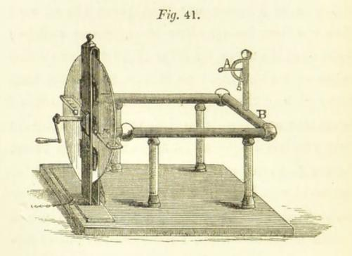
machine arranged for the purpose of rubbing glass with silk, and for obtaining the power called *electricity*; and the moment the handle
